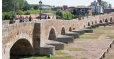
Bridge over the River Órbigo
