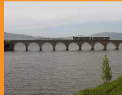
Railway bridge. Arija
