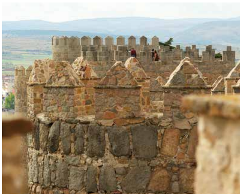
A view of Ávila's city walls from the battlements.
